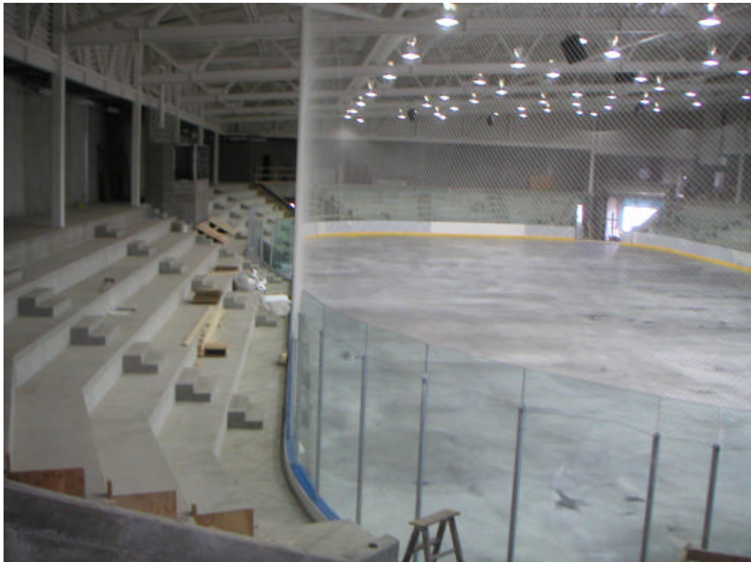
Okotoks Centennial Arena (Okotoks, Alberta)
